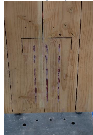
F – Finished repair ready for new fasteners
