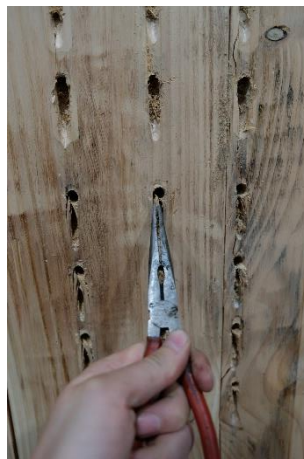
B – Removal of loose fibres with pliers
